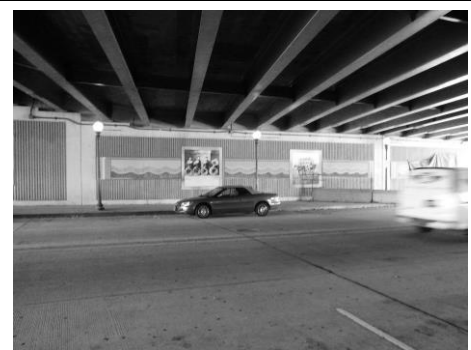
View of 8th Street SE beneath I-695
