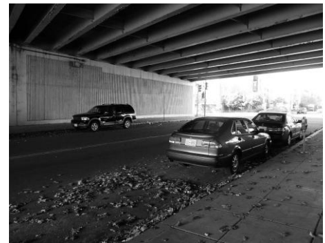
View of 7th Street SE beneath I-695
