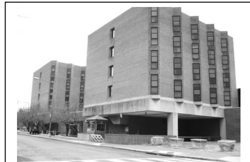
View of Building 20 below grade parking entrance and overhead berthing
