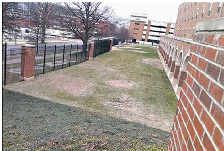
VIEW, SOUTH SIDE OF SITE AT BUILDING 25, MARCH 2014
