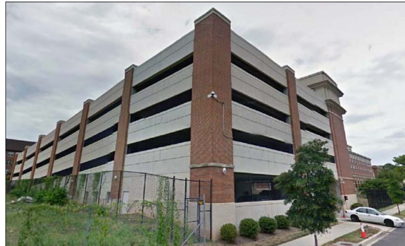
VIEW, SOUTH FACADE EXISTING CONDITIONS MAY 2014
