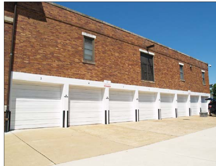
GARAGE AT BUILDING 7, MARCH 2014
