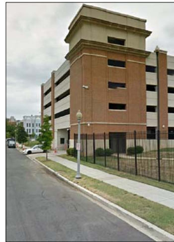
VIEW, SOUTHEAST CORNER EXISTING CONDITIONS MAY 2014
