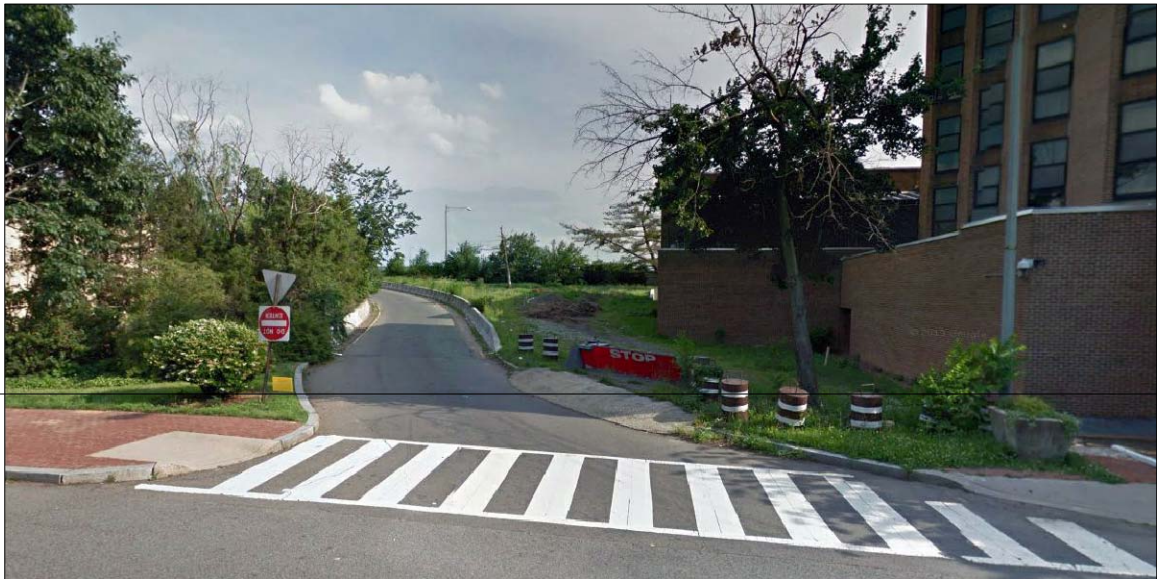
BUILDING 20 EXISTING FREEWAY ACCESS RAMPS 2014
