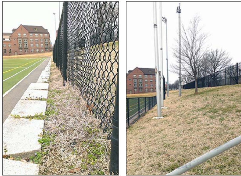
VIEW, NORTH SIDE OF SITE, AT RECREATIONAL FIELD, MARCH 2014
