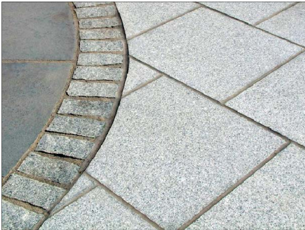
MAIN GATE DRIVEWAY PROPOSED SOLUTION: REPLACE EX. SETTS WITH SAWN FLAMED SETTS Image: comparison, hewn granite (left), sawn flamed granite (right)
